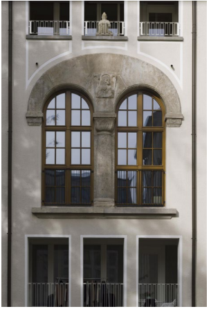
» 2009_Hild und K - Kloistergarten-Lehel » A residential development reusing the windows of a collapsing monastery. Continuing the heritage of the building(elements).
