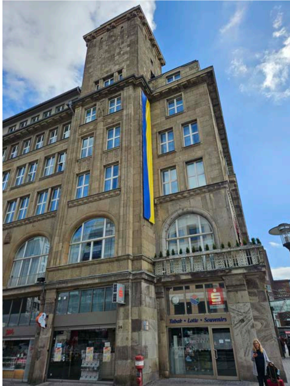
Representative "exterior" facade
