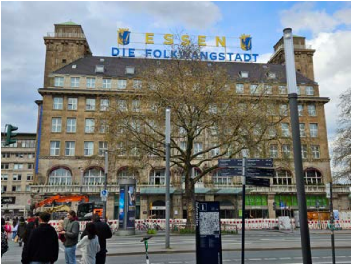
View from the station square towards the building
