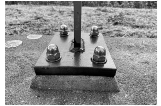
Steel footplate with bolts
