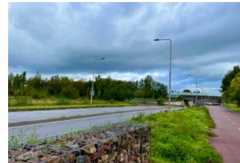
3. Infrastructure The road and railway form a dividing line; the bike lane serves as a connector.
