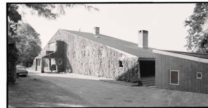
73. McKim, Mead and White, Low House and Guesthouse, Bristol, R.I.
