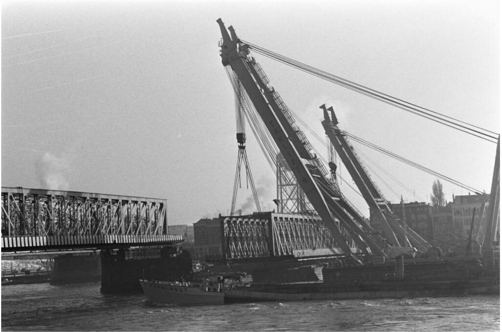
Demolishing the bridge in 1981
