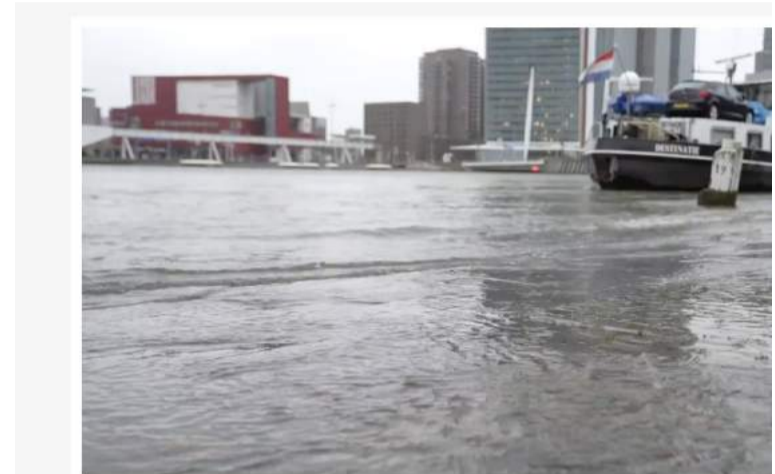
flooded quay, noordereiland source: AD
