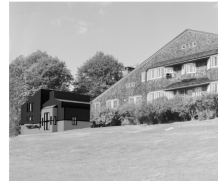
96.1 McKim, Mead and White, Guest House and Low House, Bristol, R.I.
