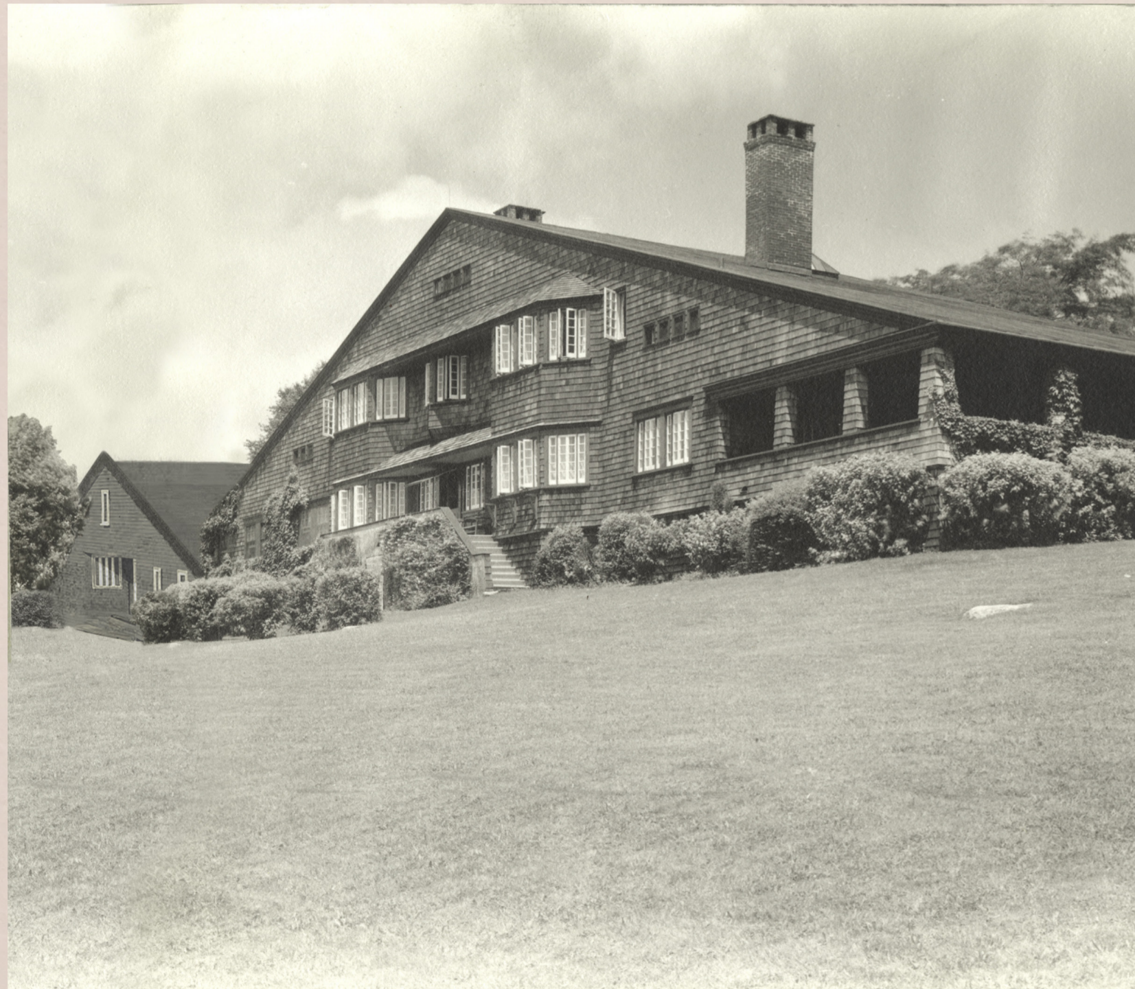
159. The Low House's guest house, which stood behind the Low House itself, 1907
