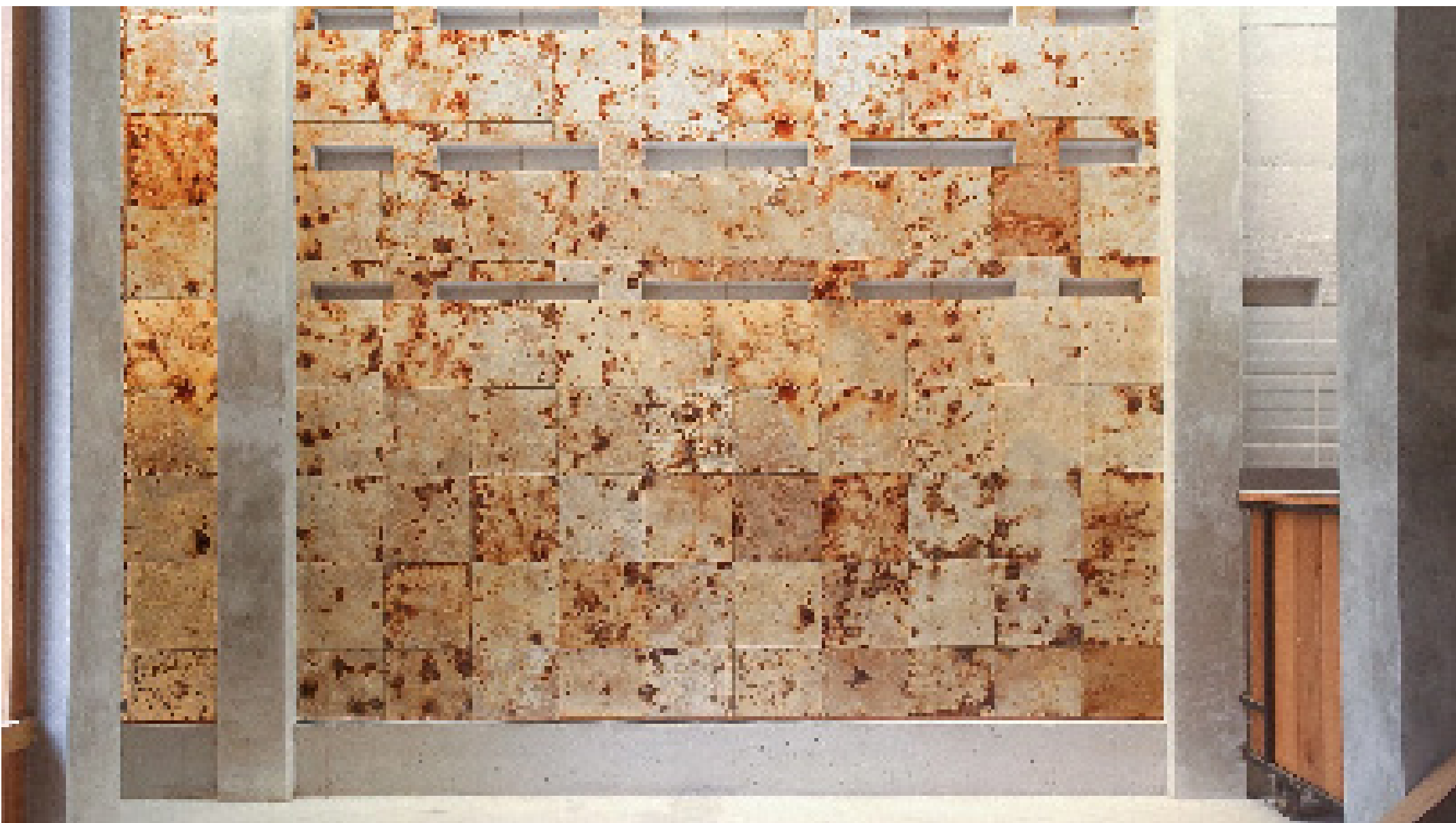
KIT, ETH, and FCL Mycelium construction panels
