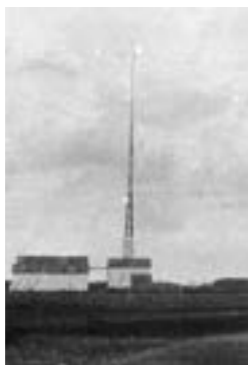
MN7 - transmission tower WO1 Technological
