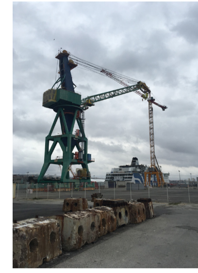
A continuous process of (re)use: industrial structures are not only a physical double, but also a layer of history
