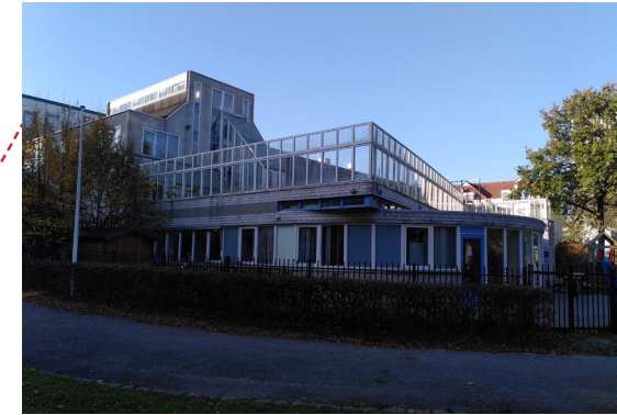
Detail building back
