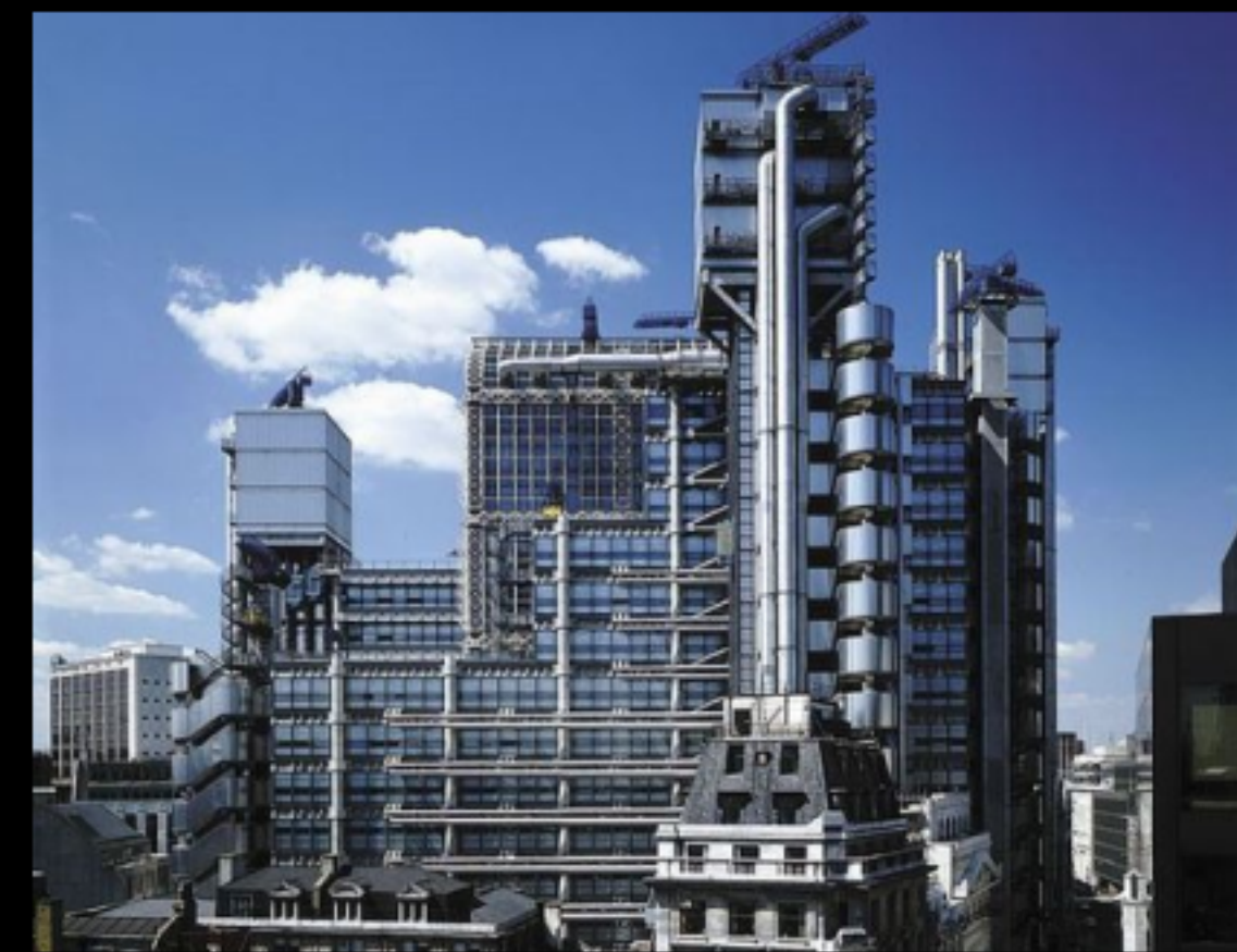
Lloyds Building, London
