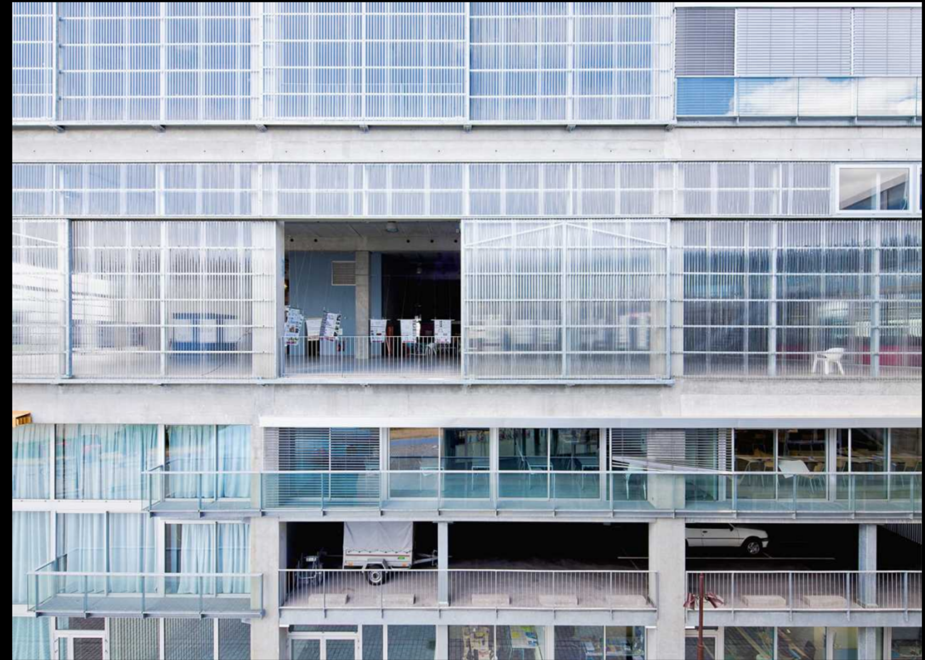
Lacaton & Vassal, Nantes School of Architecture
