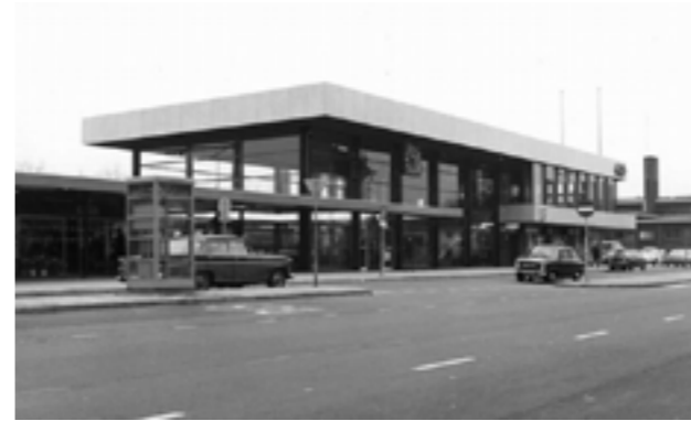
1971 | Station Bergen op Zoom, Architect Cees Douma
